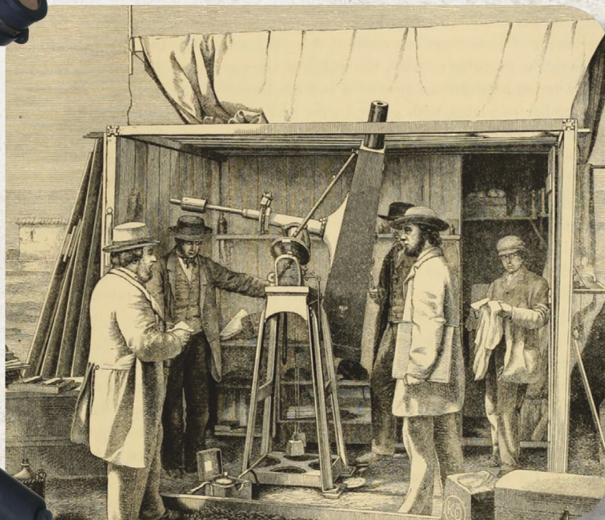
▲ THE ECLIPSE OBSERVATORY Warren De la Rue and his assistants gather around the Kew photoheliograph. The front wall of the shed was removed to take this photo. De la Rue is on the far left. The doorway on the far right leads to the darkroom.
