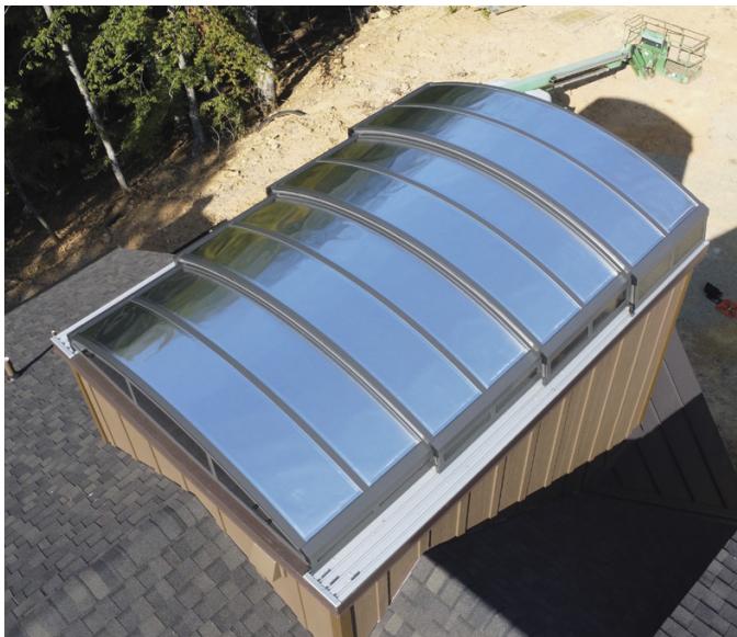
▲ INNOVATIVE REPURPOSE Left: The segmented roof panels of the observatory are a commercial product designed and marketed as retractable pool, spa, or outdoor bar enclosures but serve as excellent roll-off roofing. Right: Overlapping rubber skirts prevent rain or moisture from entering the building when the roof is closed. The folding stair enclosure’s cover is visible to the right of the pier.
