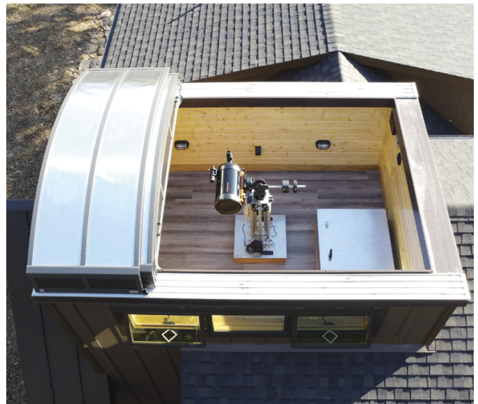
▲ INNOVATIVE REPURPOSE Left: The segmented roof panels of the observatory are a commercial product designed and marketed as retractable pool, spa, or outdoor bar enclosures but serve as excellent roll-off roofing. Right: Overlapping rubber skirts prevent rain or moisture from entering the building when the roof is closed. The folding stair enclosure’s cover is visible to the right of the pier.
