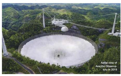
THE RADAR SYSTEM at the Arecibo Observatory in Puerto Rico was once the most powerful source of electromagnetic radiation on this planet, enabling the mapping of Venus, the Moon, and near-Earth asteroids. Then, in 2020, support cables for the giant dish's observing platform failed, resulting in the collapse and permanent closing of the storied telescope (S&T: Mar. 2021, p. 8). Now, an inquiry has found those very radar transmissions may have helped trigger the collapse.
