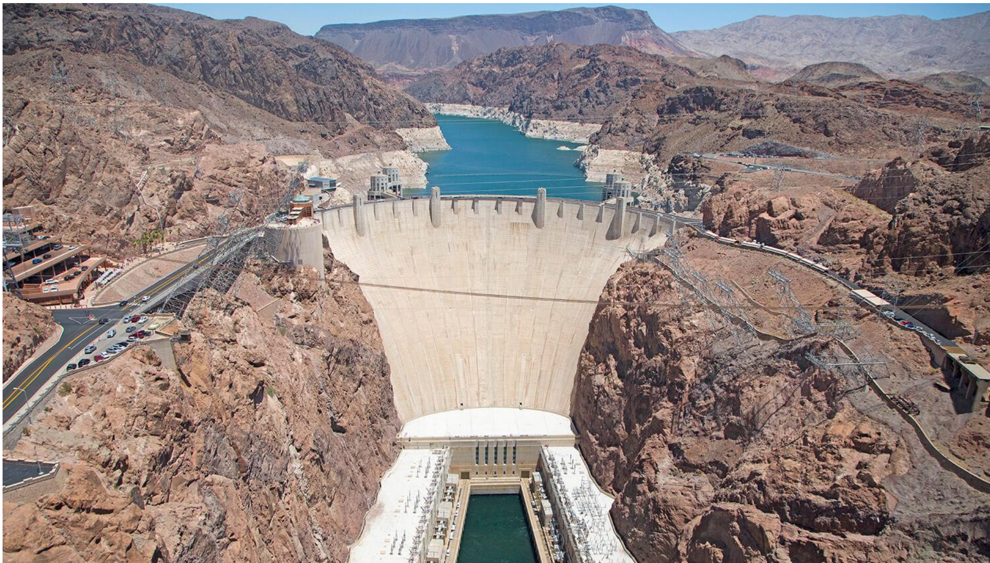
Hoover dam (Colorado river)
