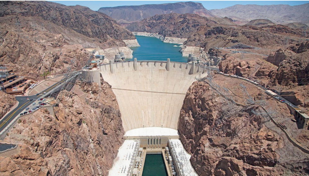
Hoover dam (Colorado river)
