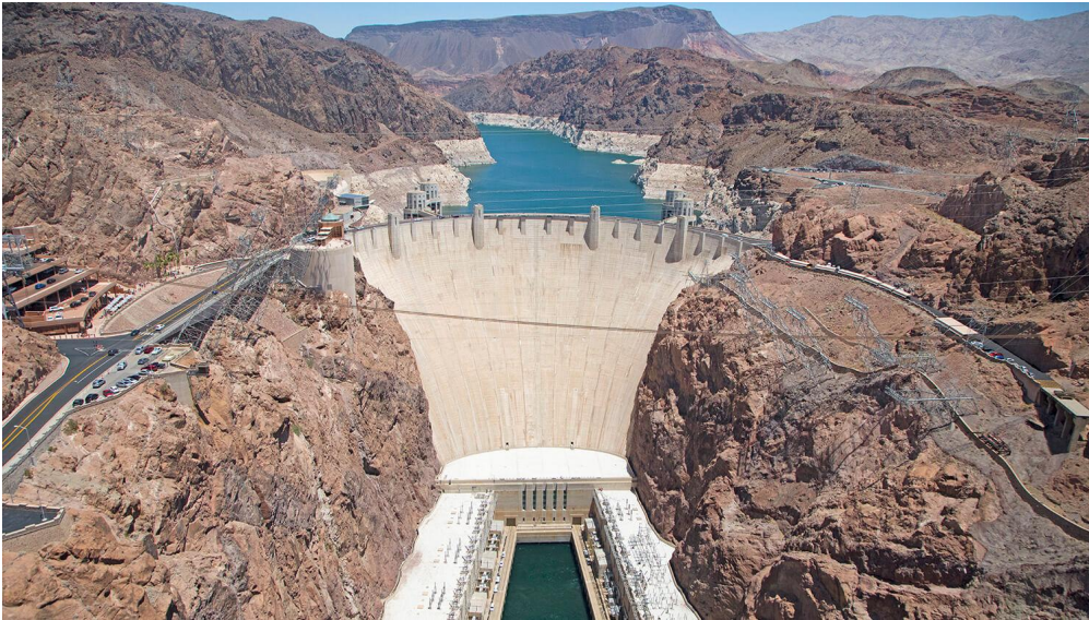
Hoover dam (Colorado river)
