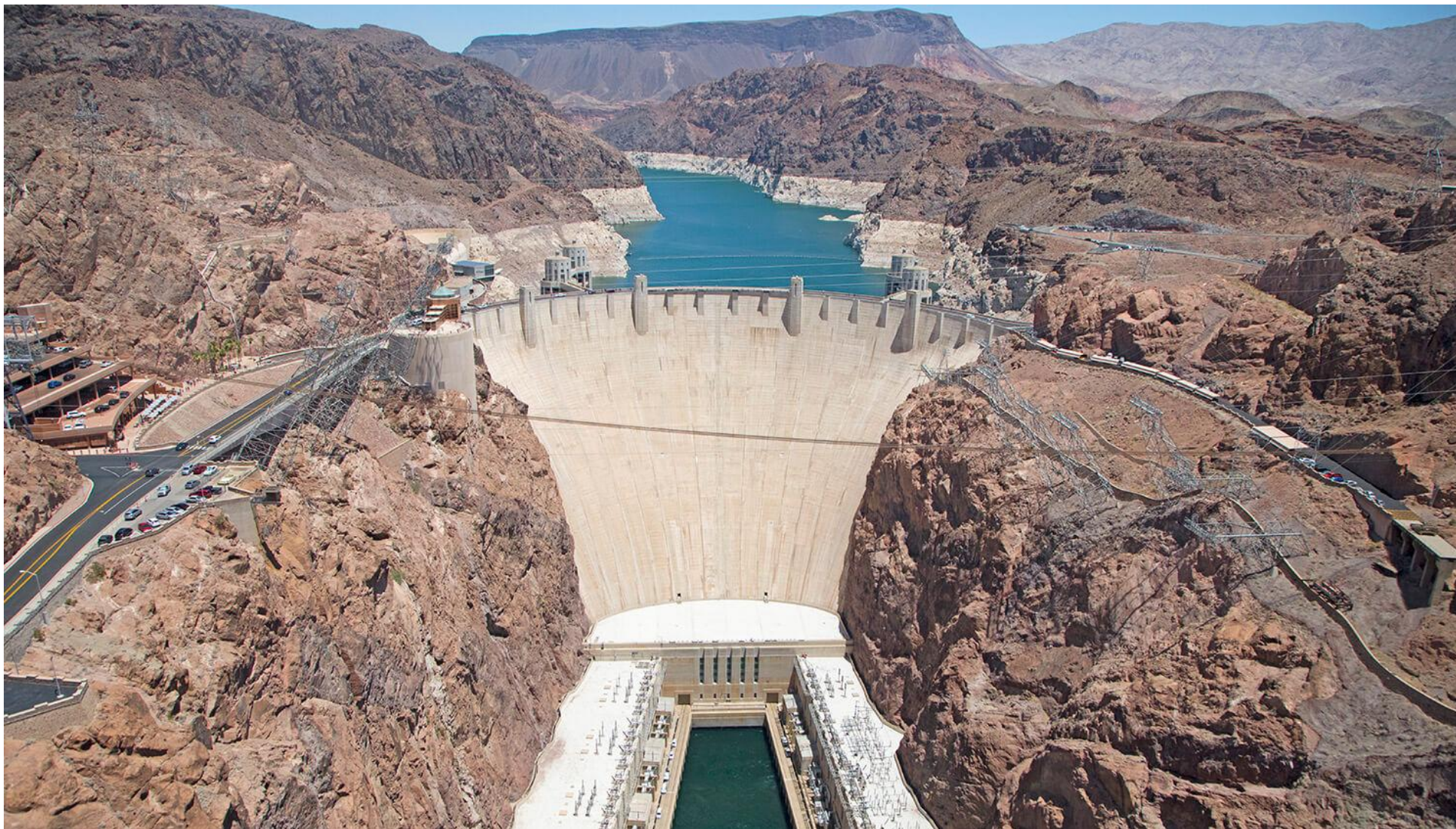
Hoover dam (Colorado river)
